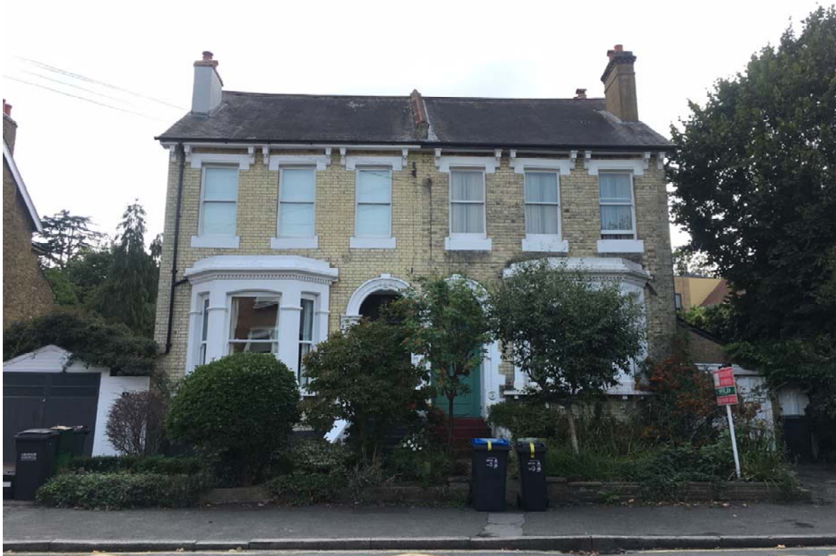
Fig 2: Photo of the semi-detached pair with the subject site on the right hand side
